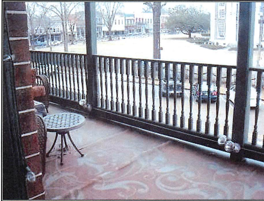
Viewing balcony of subject building
