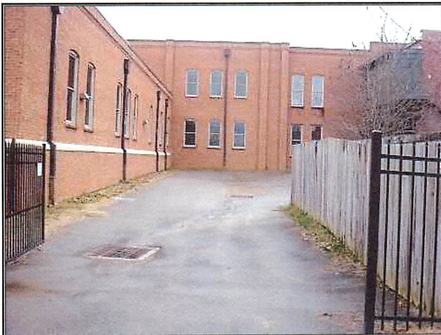
Viewing east across rear parking area from Union St.
