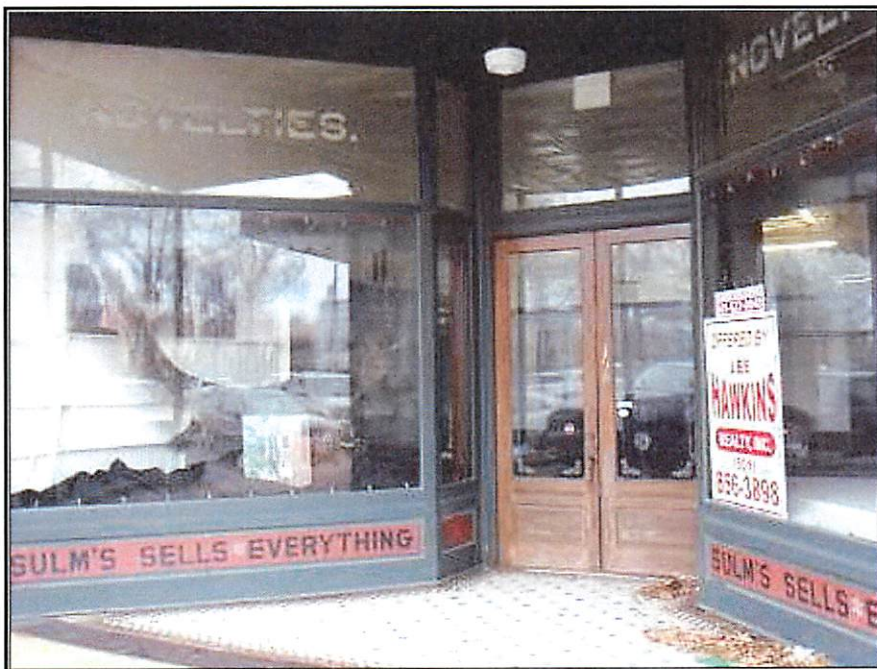
Viewing front main entrance to subject building
