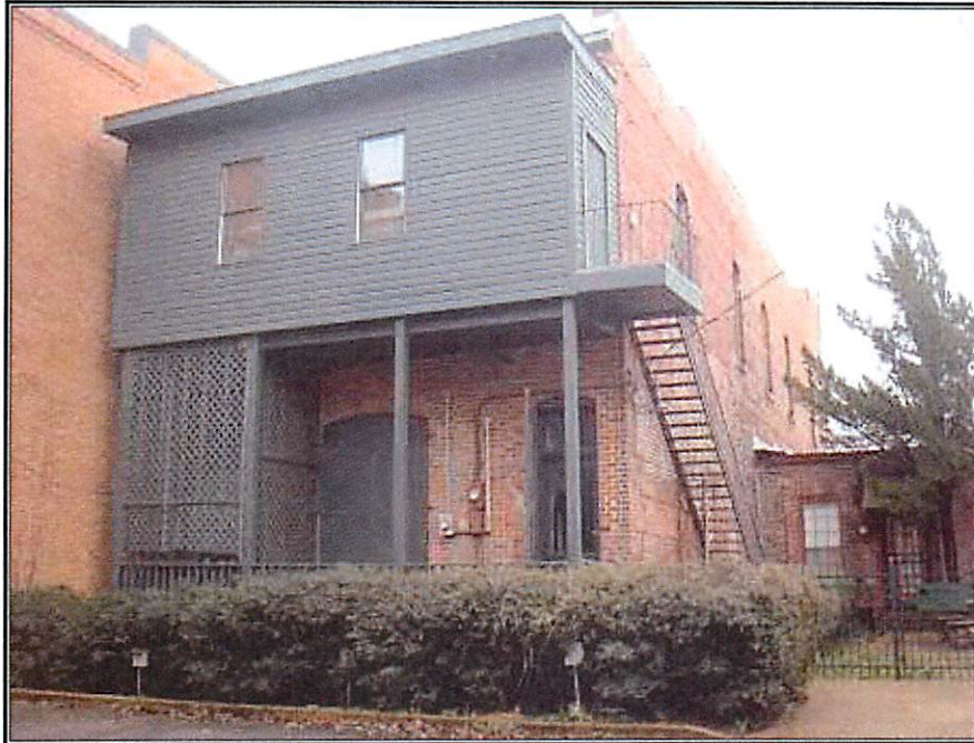
Rear/side view of subject building from rear parking area
